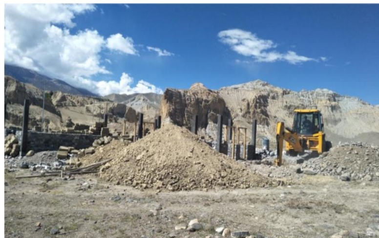
Pillar standing and digging septic tank
