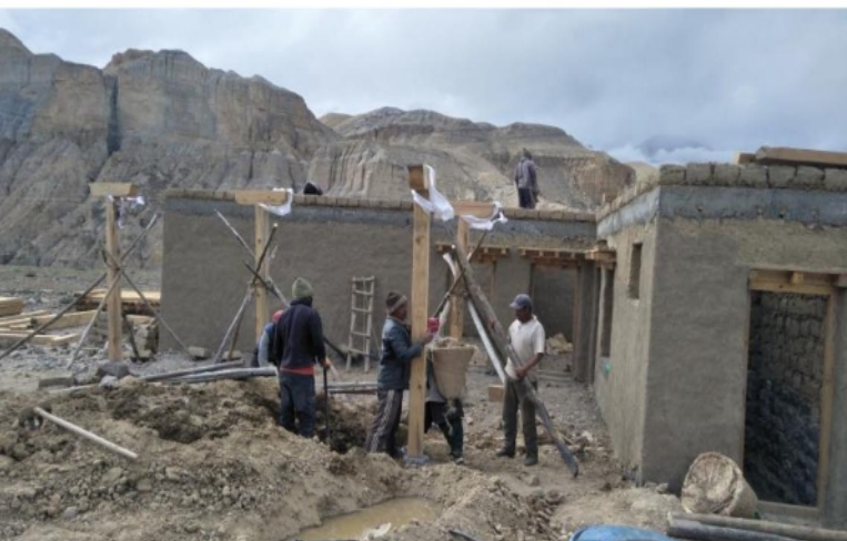
Pillar standing and digging septic tank
