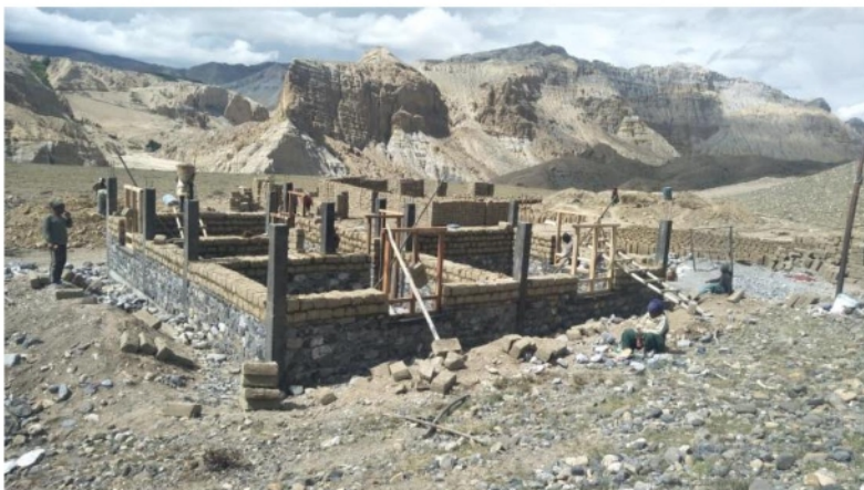
Clay Mud Brick for house wall construction
