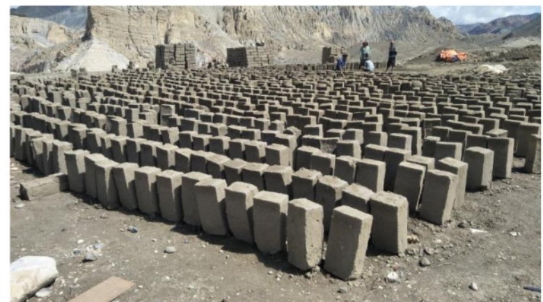
Clay Mud Brick for house wall construction
