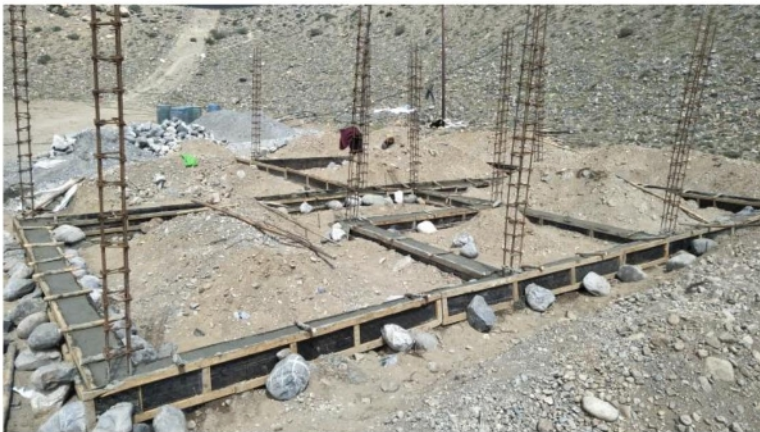
Foundation construction of health center
